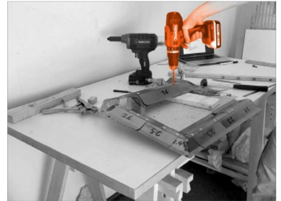
② pre-drill rivet holes
